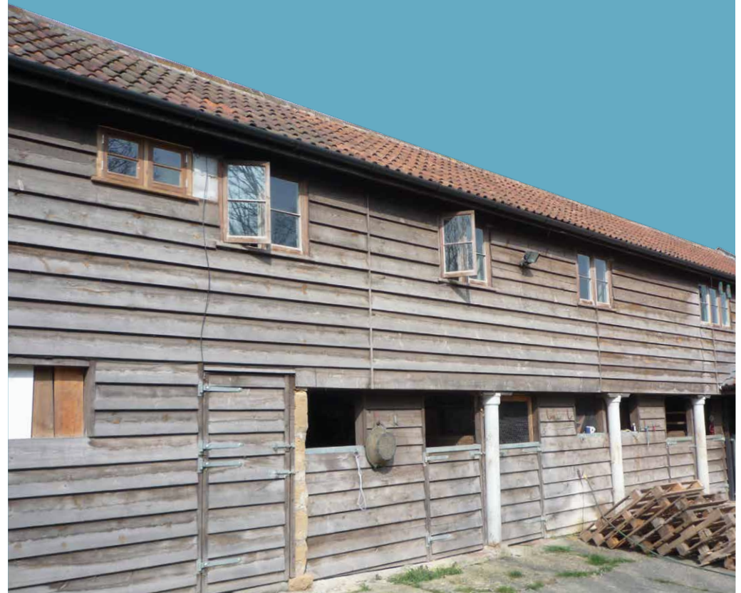
Linhay style building in Combe Hay
